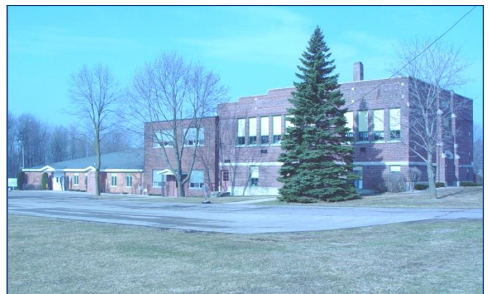
1925 with additions in 1954 and 1968
